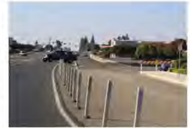
SR108 has many sections with significant unused right-of-way area ideally suited for LID treatment facilities.
