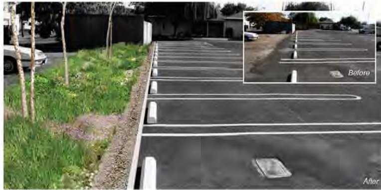
Filter strips can be as simple as a gentle slope covered in grass that receives runoff from an adjacent strip of parking stalls.
