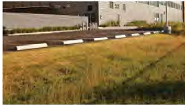
Filter strips can be as simple as a gentle slope covered in grass that receives runoff from an adjacent strip of parking stalls.
