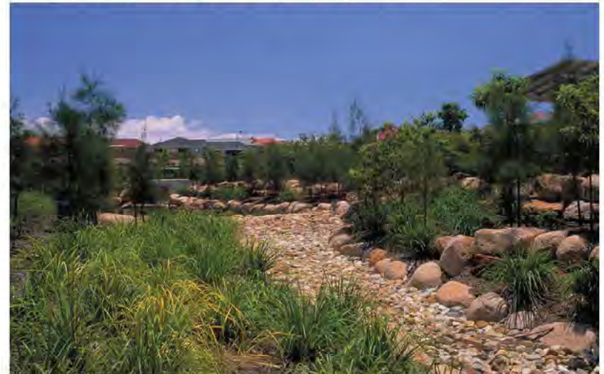
The deployment of BMPs on a site can take many forms, which allows the facilities to integrate with landscaping while still providing optimal stormwater functionality. These examples show bioretention areas within an outdoor courtyard (above left), a vegetated swale and filter strip serving as a buffer for homes (above right), and a rocky swale area meant to be appealing while dry but able to handle infrequent large flows.
