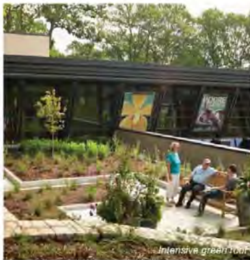
Intensive green roof
