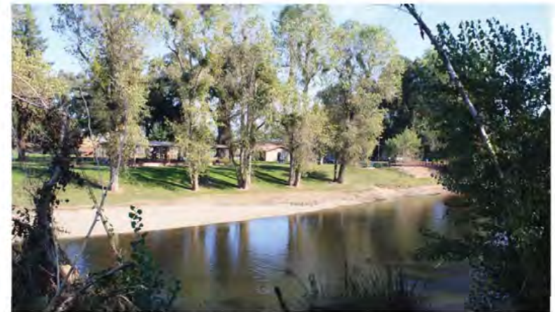
Jacob Meyers Park, located adjacent to the Stanislaus River, has numerous structures and development located within the floodplain.
